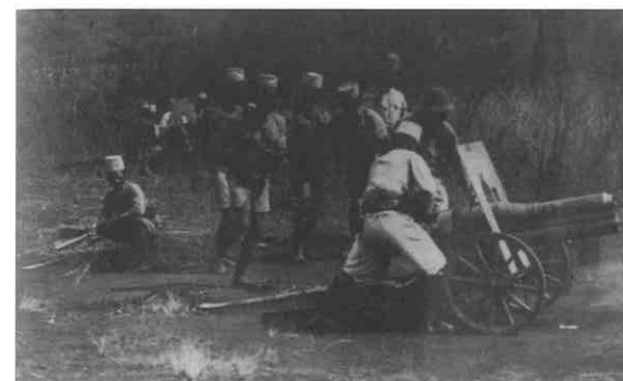
Belgian Force Publique gunners firing a French-supplied 70mm St Chamond mountain gun. This piece could be broken down into five parts and manhandled through the bush, the trail alone requiring five or six porters. (Musée Royale de l'Armée)
