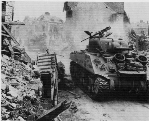
Only campaign photos reveal exactly how vehicles looked in service, including markings (official and unofficial), extra equipment, and field modifications. Here we see road wheels, track sections, and a metal box (all held in place by a length of angle stock welded across the fenders) being used as "soft" armor on a British Sherman.
