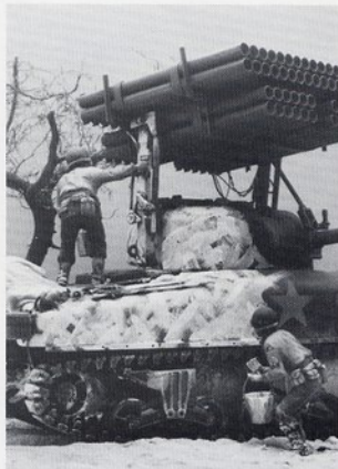
The winter camouflage being applied to this Sherman is whitewash, done in a semi-covering pattern suited to wooded terrain. Units in the field used brushes, mops, and even rags for painting.
