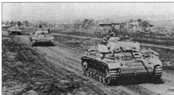
An unidentified PzKpfw III battalion passes a ruined village in the Mius-Stalino area, August 1943. The lead vehicle has a turret-girdle of spaced armour but appears to carry side-skirts on the far side only. (Bundesarchiv)
