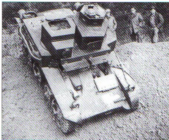
The final production batches of the M2A2 light tank used slab-sided, welded turrets as can be seen in this overhead view of a tank on maneuvers at Fort Belvoir, Virginia, on 22 November 1940. (US Army MHI)
