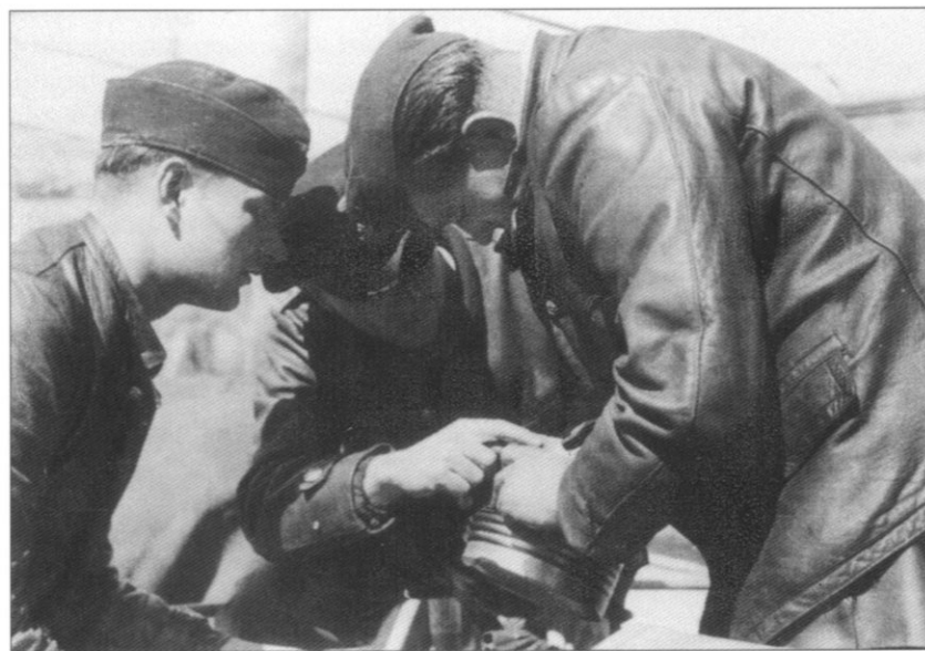
Engine room crewmen performing maintenance on one of the diesel engines. One of the pistons has been removed for examination as the 'Chief' points to an area of damage. Major repairs usually required the removal of the engine from the boat.
