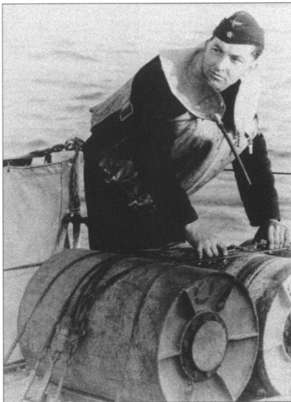
A crewman in life jacket checks the depth charges carried on his boat. Normally, when loaded, three charges were carried in each of two stern racks.
