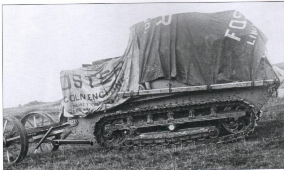
Draped with tarpaulin covers disguise its warlike purpose, the Lincoln Machine is shown during trials. This photo was taken after the tracks had been modified, but they still proved unsuitable for the work they would have to do.
