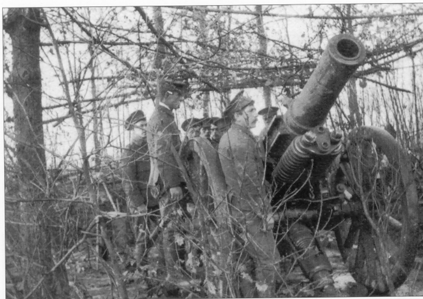
BL 6-in. 30cwt howitzer of 6th Siege Battery, RGA, 1914-15. The large buffer springs of the BL 6-in. 30cwt are clearly shown in this photograph, as is the arm and volute spring linking the howitzer to its siege platform. (RAHT AL190.3.28)
