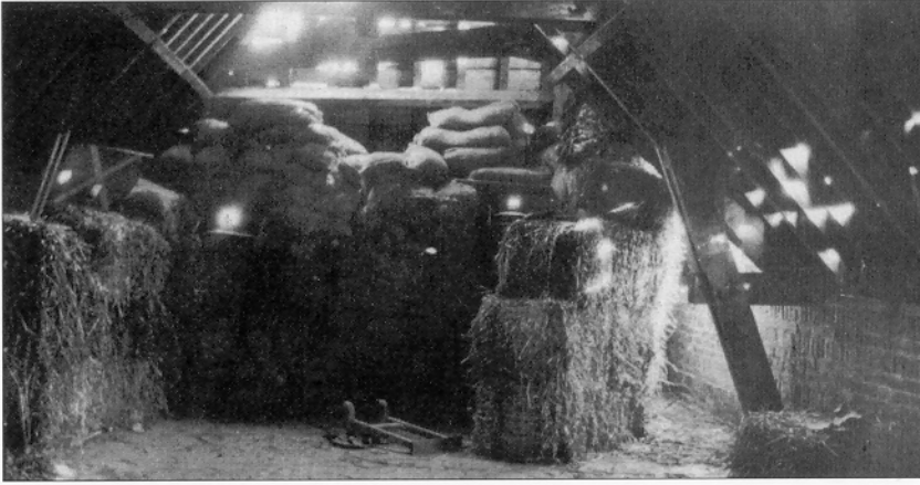
Interior of a primitive OP in a barn at Precepteur, Foucaucourt, October 1915. Sandbags and hay bales have been arranged to give protection. (RAHT AL445.56)
