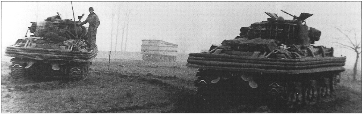
DD tanks of the Staffordshire Yeomanry, already veterans of the Scheldt battles, prepare for the Rhine Crossing in March 1945. The nearest tank shows well how neatly the screen could fold down if done with care. In the background another DD waits, with its screen partly raised.
