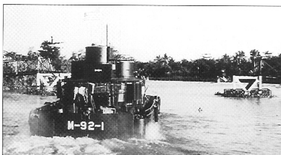
Monitor M-92-1 approaches a downed bridge. Most bridges in the Delta had been destroyed by the Viet Cong (VC). Only around major population centers where security could be provided were bridges rebuilt. The lack of rural bridges made the waterways even more important for commercial transportation.
