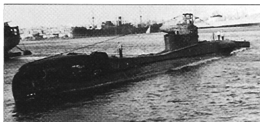
The successful T-Class HMS Turbulent was lost with all hands in March 1943, the dead including its famous commander J. W. 'Tubby' Linton, VC. Note the aft-pointing external tube behind the conning tower.
