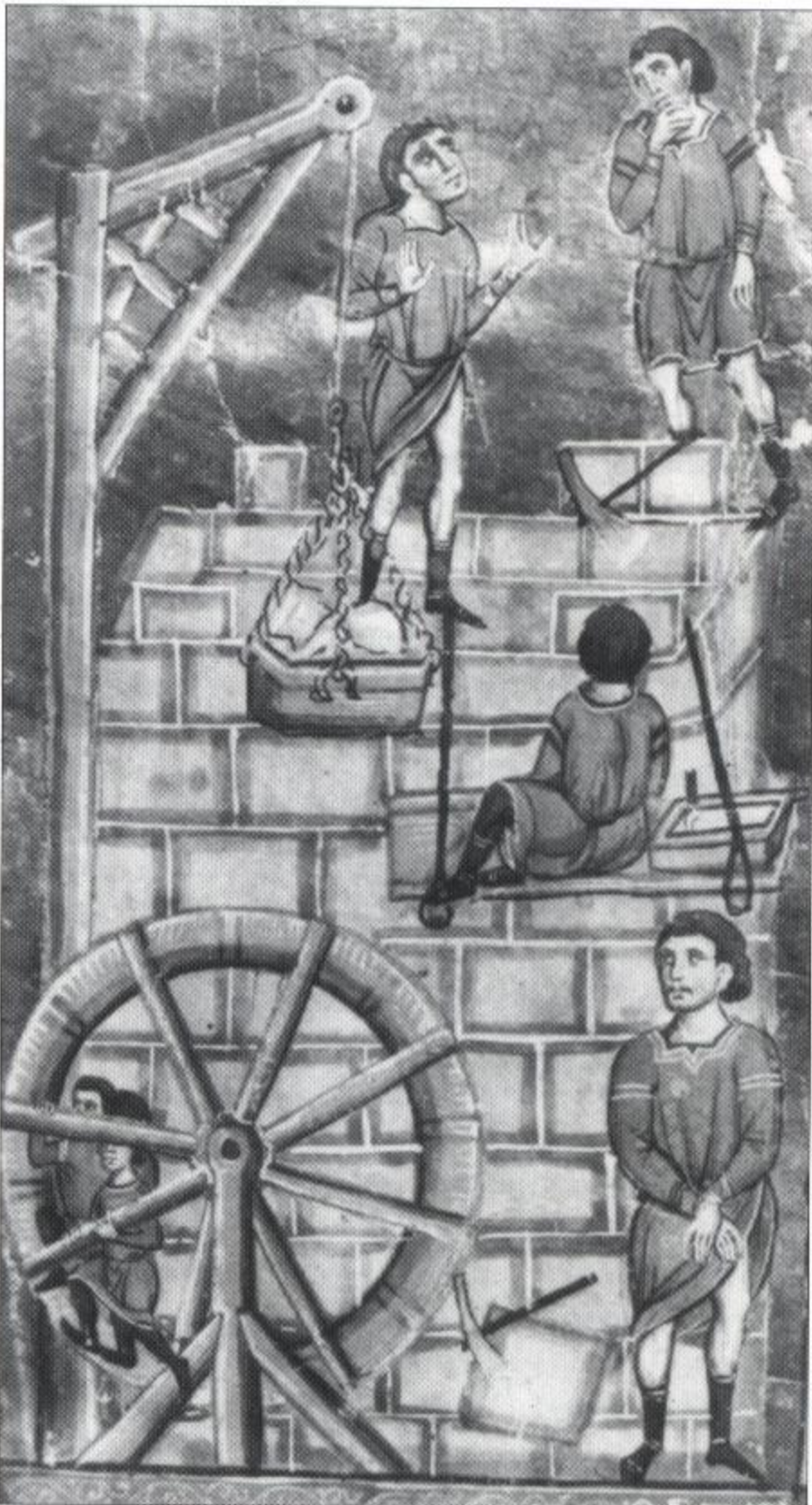
BELOW 'Tower of Babel', Universal History of William of Tyre, Acre, late-13th century. The labourers wear clothes in a mixture of western, Byzantine and Islamic styles while building techniques include a typical Middle Eastern mould for making unbaked mud-bricks. (Bib. Munic., Ms. 562, Dijon, f.9r)
