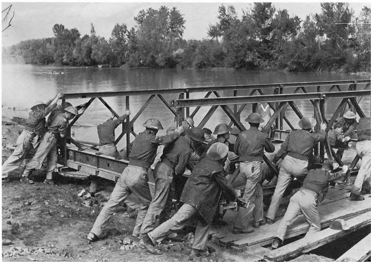
20 Sappers launching a Bailey bridge in Italy. This invention, together with the armoured scissors bridge which was also used by the divisional RE, proved invaluable in NW Europe, where most of the bridges over the numerous rivers and canals had been blown. (Imperial War Museum)
