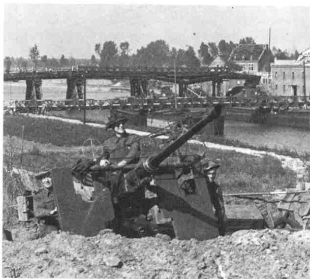
A familiar task for the 40mm Bofors guns of 94th LAA Regt., RA: guarding Bailey bridges built by the sappers on the divisional or brigade centre lines. The nearer bridge has been spanned across moored civilian barges, while under the further one trestles have been built to replace the blown piers of the original masonry bridge.
