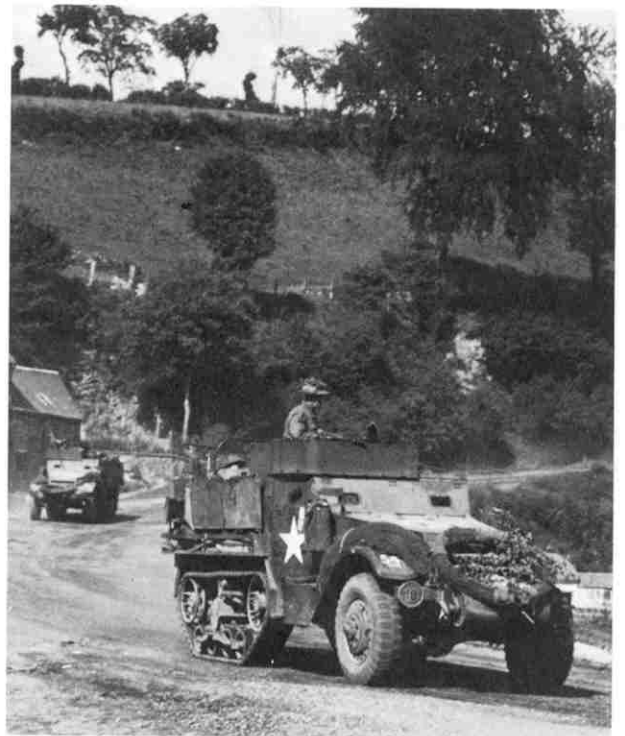
M3 halftracks of 1st Motor Bn., Grenadiers. The unit tacsign—'54' on red—the ground and air recognition stars, and the bridging circle—yellow rim, black '10' outlined in yellow on circular khaki plate—can be seen on nearest vehicle. These are the motor infantry version of this vehicle, used by many units within the Division in different forms. Each carried one section, and had a ring for an AA machine gun beside the driver, side racks and hoops for rigging a canvas tilt over the open body. Rolls of barbed wire were often carried on the front as here.
