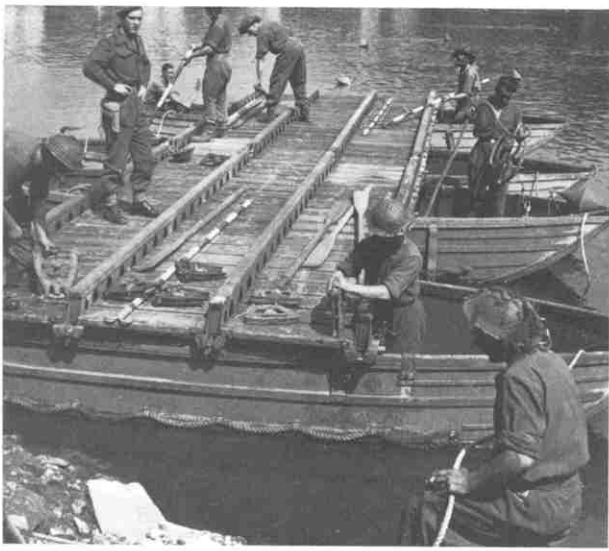
Sappers building a pontoon bridge with folding boat MkIII equipment. This could take light loads such as cars, but the stronger Bailey bridges were used on the main axes and centre lines where bridges up to class 40 specification were needed for the tanks.
