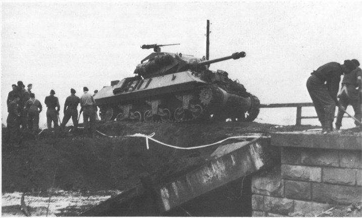
The last lap. Airborne Engineers repair a blown bridge for the passage of an Achilles tank destroyer: Coesfeld, 30 March 1945. (Imp. War Mus.)
