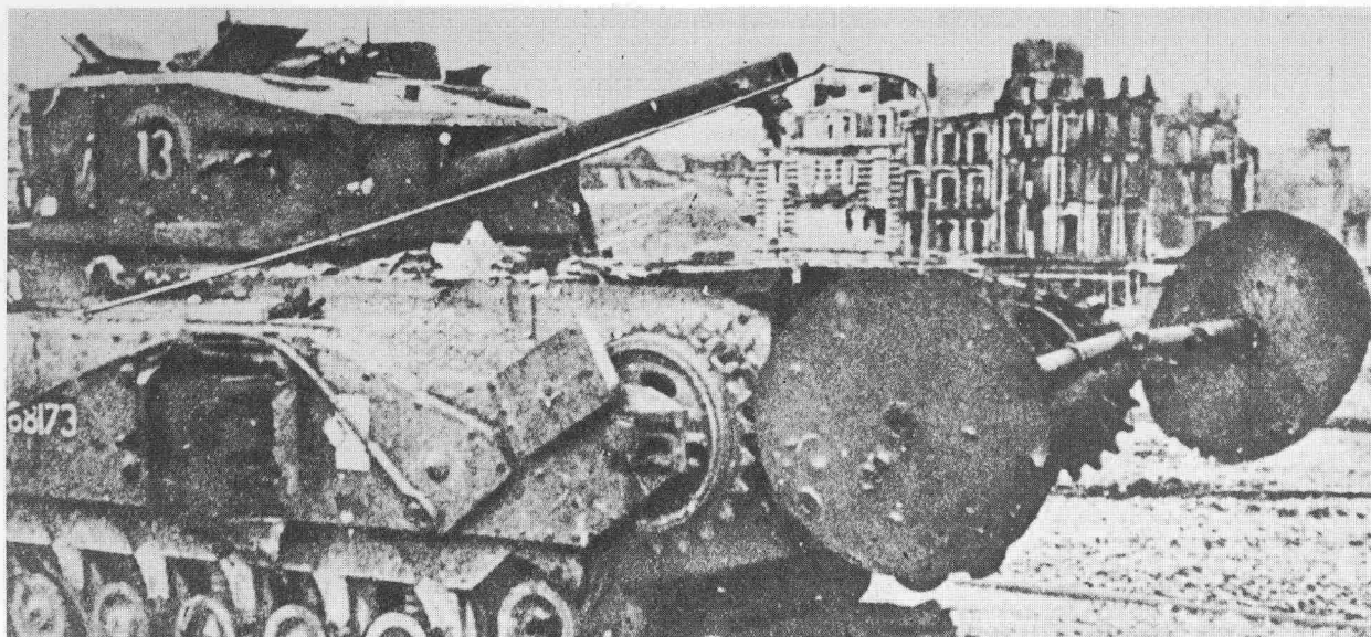
One of the tanks to cross the sea wall was this 'C' Sqn. Mark III carrying an elementary bobbin mat-layer.
