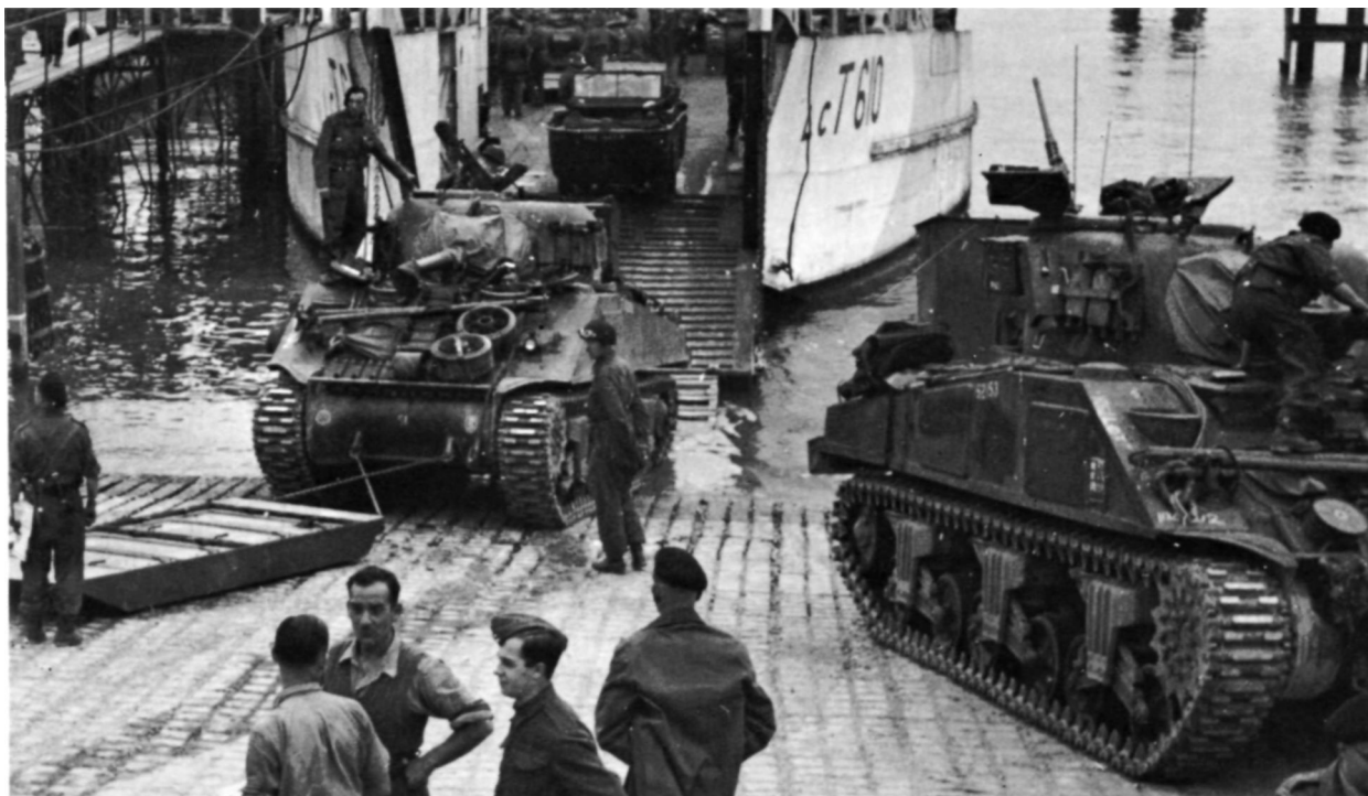
Loading for the invasion of North-West Europe. Waterproofed Shermans of 13th/18th Hussars, 27th Armoured Brigade, reversing into a Landing Craft Tank at Gosport in June 1944. The smaller LCTs carried the assault waves of tanks while the larger LSTs brought in the follow-up waves once the beach was empty.
